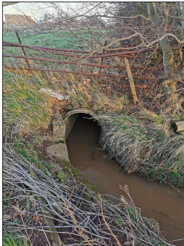
Figure 4 – Old A1 / Skateraw culvert entry (900mm concrete pipe)
