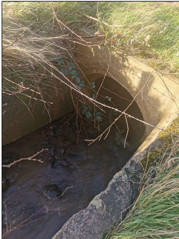
Figure 2 – A1 culvert entry (900mm concrete pipe)
