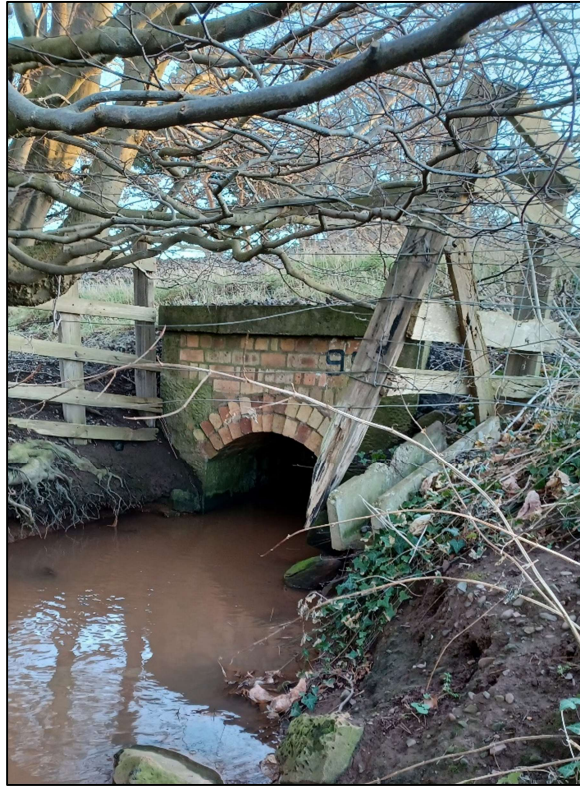
Figure 3 – Railway culvert exit (1000mm wide concrete / brick lined arch culvert)
